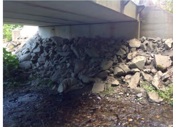
Right Bank Abutment when facing downstream
