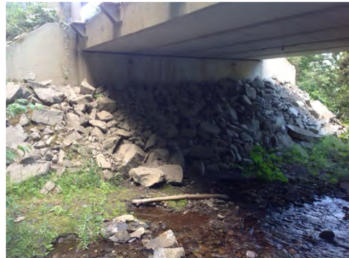
Left Bank Abutment when facing downstream
