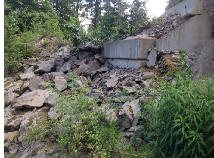
right bank downstream wall
